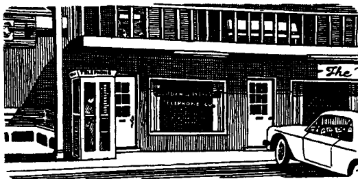
Business Office of the Continental Telephone Company of California overlooks the park in the central section of Kernville. The office serves the entire Kern River Valley region.
